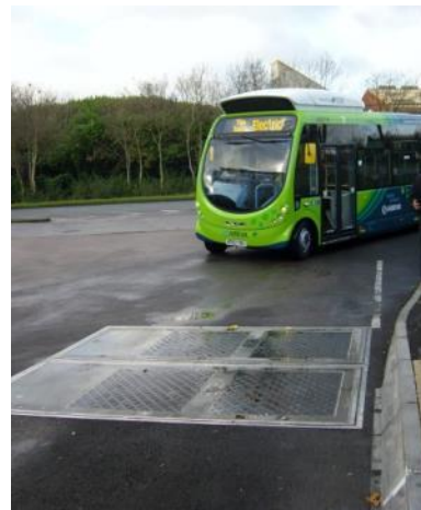
Figure 5: A Milton Keynes electric bus approaching an inductive charging pad.
