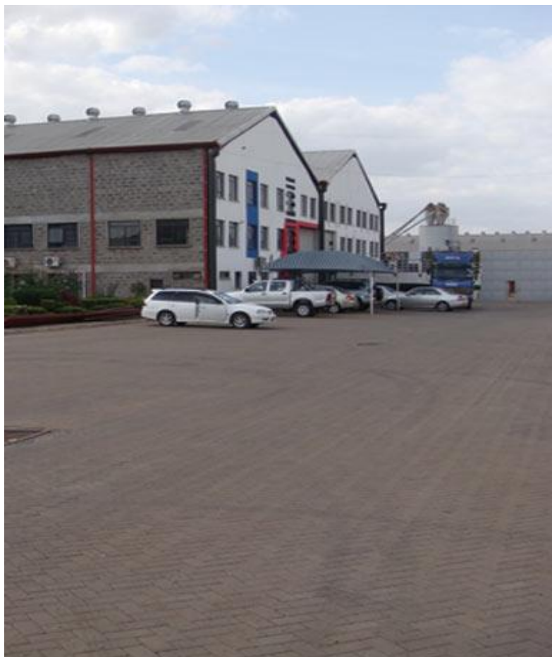
Figure 5.6: Premises of a highly formal sector firm
