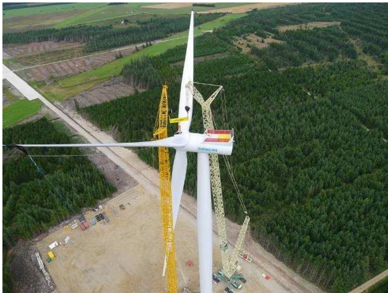
Siemens WP 6 MW DD turbine installation
