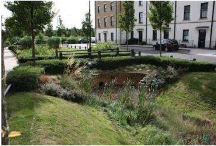
Figure 3 An illustration of the use of a swale in managing exceedance flows – a network of swales conveys flows in excess of the 1 in 30 year design event safely through the Upton housing development (Ciria)
