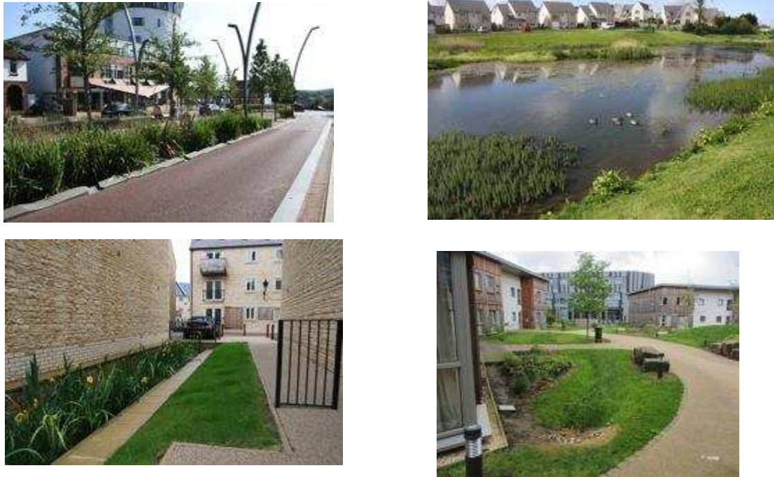
Figure 1 Examples of SuDS schemes – clockwise from top left: Highway draining Biofilters in Ashford (Sue Ilman); Storage basin Hamilton (Brian D’Arcy); University of York campus swale (by permission of Arup); Linear wetland, Stamford (Steve Wilson)
