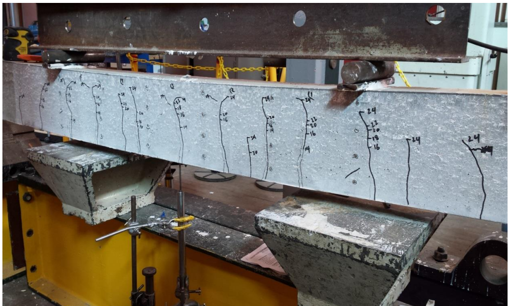
Figure 6-9 Crack pattern of the steel reinforced concrete beam.
