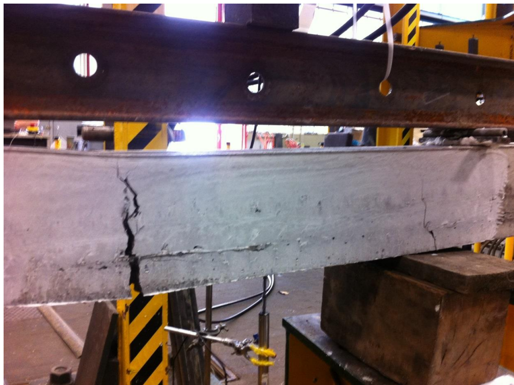
Figure 4-30 Cracks patterns of BT (5cm) 14-Anch-2.6-L, 50k
