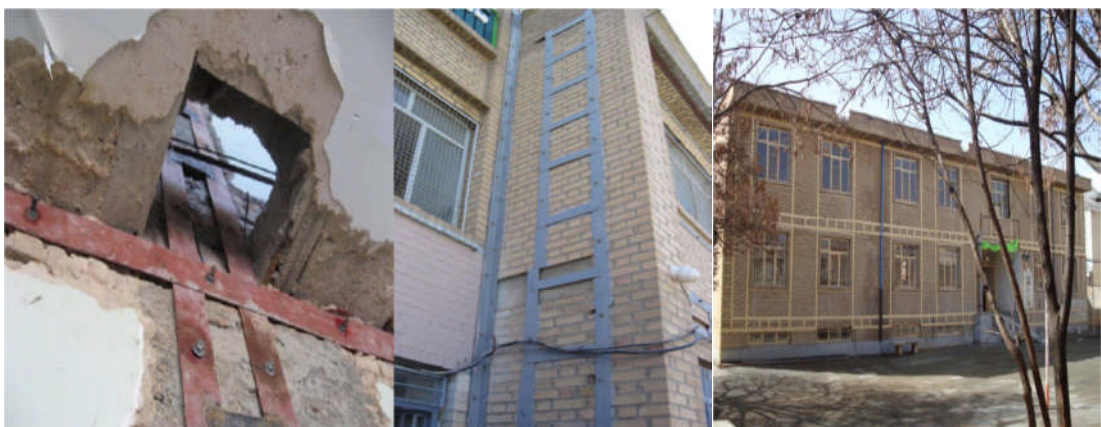
Figure 2.4 – Steel strapping the masonry walls in schools (SRO 2011)
