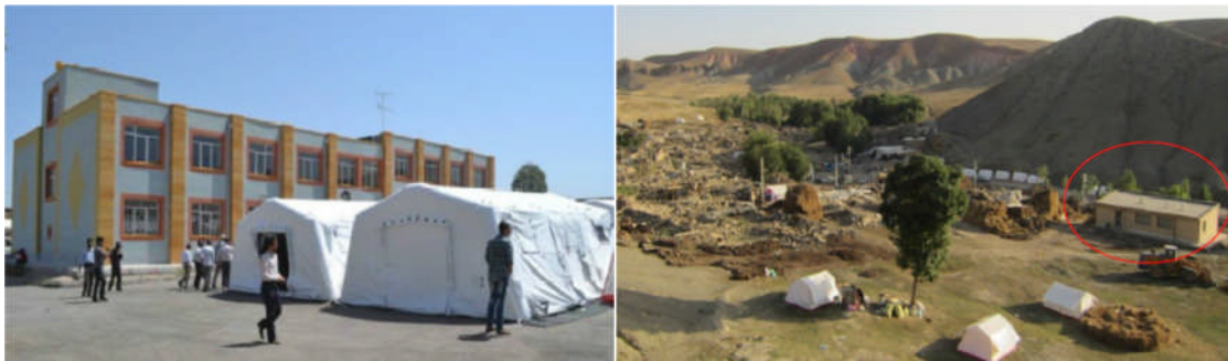
Figure 2.5 – The new retrofitted schools survived and served after an earthquake (SRO 2011)
