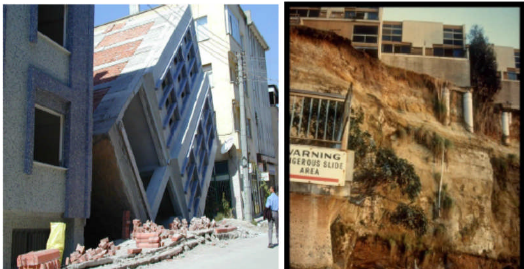
Figure 6.10 - Liquefaction and sliding hazard in Kocaeli, (Turkey 1999) and Loma Prieta, (Mexico 1989)
