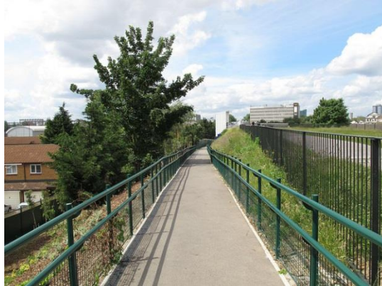
Figure 3.6: New access ramp to the Greenway (Craven, 2012)
