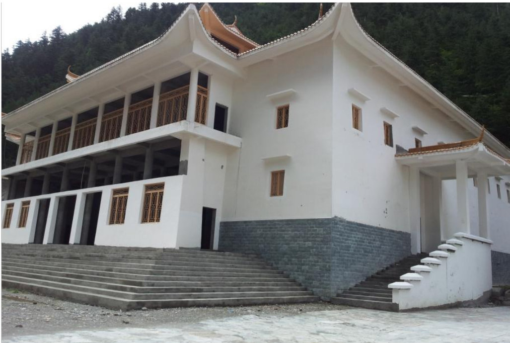
Figure 3.10 The new temple in construction
