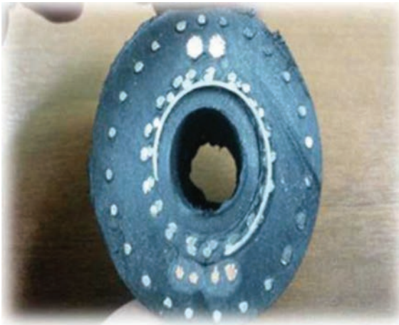
Fig. 6. Cross-section of the cable with hydraulic channel and power and signal cores
