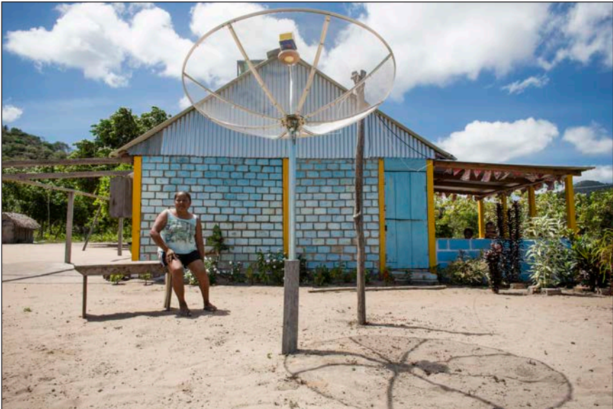
Figure 15.—Annai, North Rupununi. Houses are increasingly built using imported materials.
