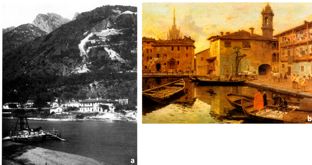
Figure 10. (a) Candoglia pier (late XIX–XX century). (b) Navigli di Milano during the Duomo di Milano construction activities (portrait). (Veneranda Fabbrica Historical Archive).
