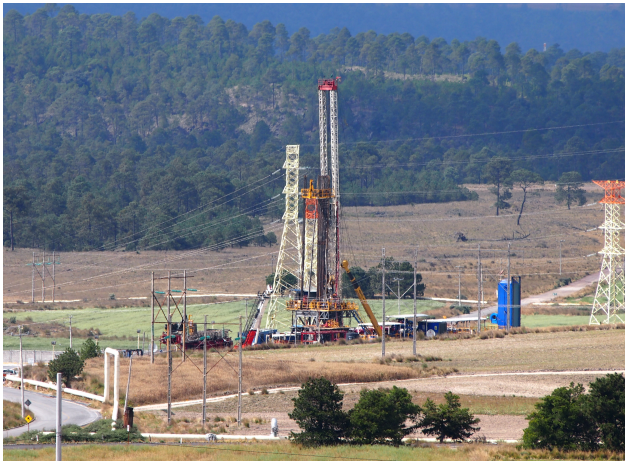
Figure 1: A drilling rig operating at Los Humeros.
