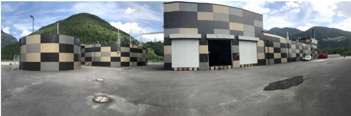
Fig. 2.1: the Wipptal AD plant (Vipiteno, BZ)
