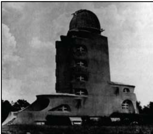
Fig. 10: Einstein Tower, near Potsdam, Germany, 1920 (Trachtenberg and Hyman, fig. 806)
