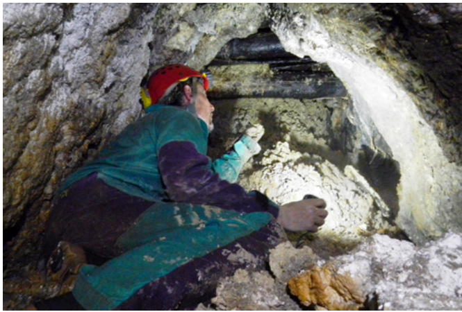
Fig. 7: view of the debris deposit, in the final sector of 3 th level gallery. This landslide block the passage to “Garbere” (photo M. Vattano).
