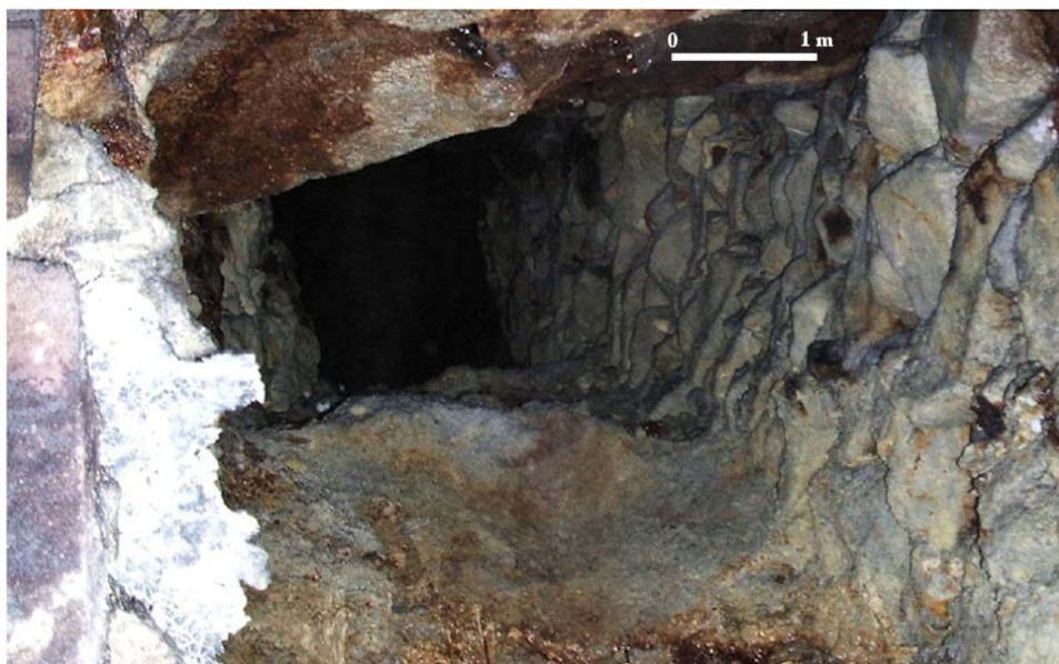
Fig. 4. Example of uplift tunnel realized into a mining fill (Courtesy of Daniele Trogolo Got)
