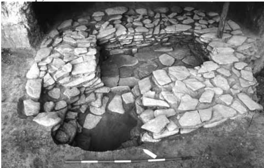
1 2 3 4 5 Fig. 2 Papillon monumental tomb (Alba-Cuneo. Northern Italy): on the left of the image you can 6 see the violation damage (sud-west corner) (From: Venturino Gambari et al. , 2011a photo CO.R.A. 7 Soc. Coop.). 8
