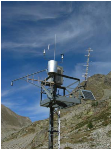
Figure 1. Spatial distribution of the ARPA Piemonte nivo-meteorological station network (a) and example of an automatic station with ultrasonic snow sensor (b).
