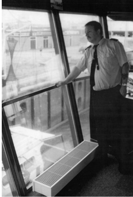
FIGURE 8. Heating radiator located exactly at the best standing position for a lock master.
