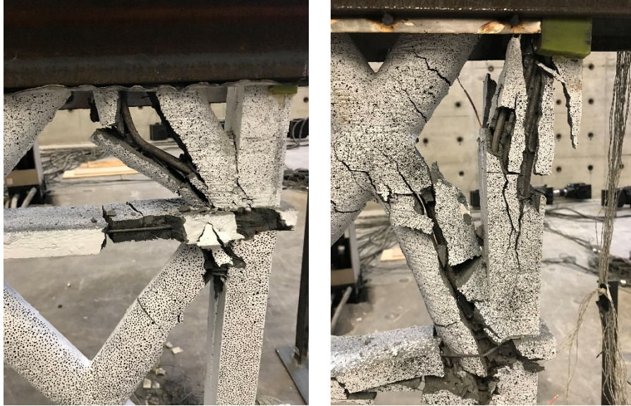
Figure 4.10: Damage observed in optimized wall at failure
