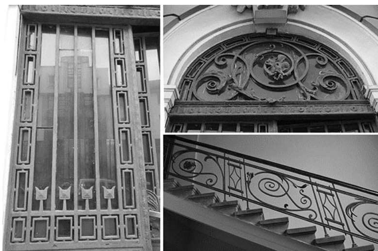
Fig. 9. Door grating, decorated window overpanel, staircase fencing in the house situated at 31, Hrushevsky Str. (1912)
