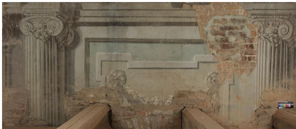
Figure 2. The area upon which the pilaster sided entablament was leaned
