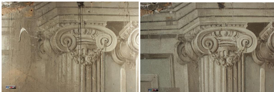
Figure 7. A detail of the wall decoration before (left) and after (right) the cleaning and conservation
