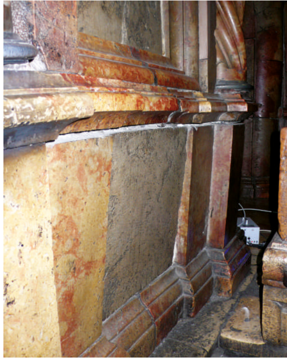
FIGURES 2A AND 2B Documentation of the Aedicula requires a high level of detail in order to record the decay and deformations of the stone.
