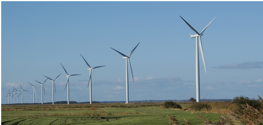
Figure 1.6: 2.3MW Siemens wind turbines in the Norrekaer Enge wind farm, Denmark [Staunited, 2018].
