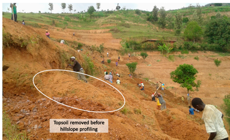
Figure 4. Practice of removing the topsoil and putting it apart before hillslope profiling during terraces implementation, according to Bekele-Tesemma, 2011 [22], Rwanda, photo of G. Castelli, 2017.
