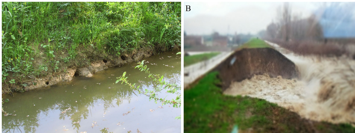
Fig. 1 a Typical burrows produced by Procambarus clarkii on irrigation ditches; b due to the burrowing activity of Procambarus clarkii broken levee alongside the river Secchia (Emilia Romana, Italy)
