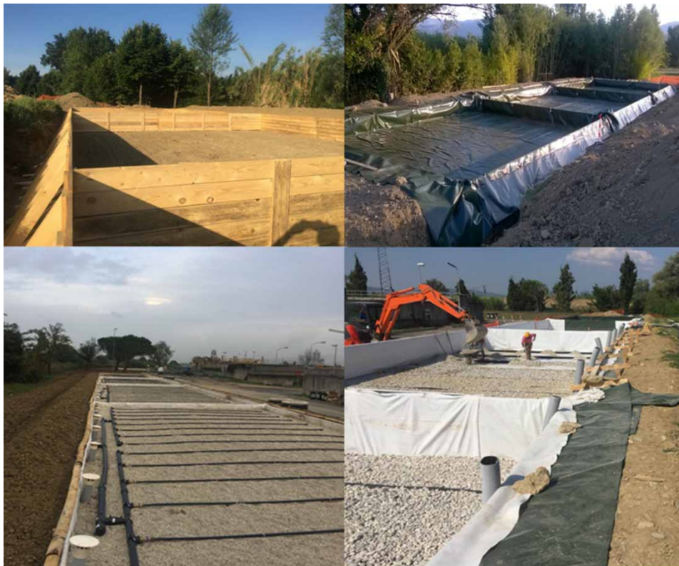
Figure 2 | Different realization steps of the pilot plant. In clockwise order: excavation and forming, laying of geotextile membrane; laying of fine gravel; inflow distribution pipes.
