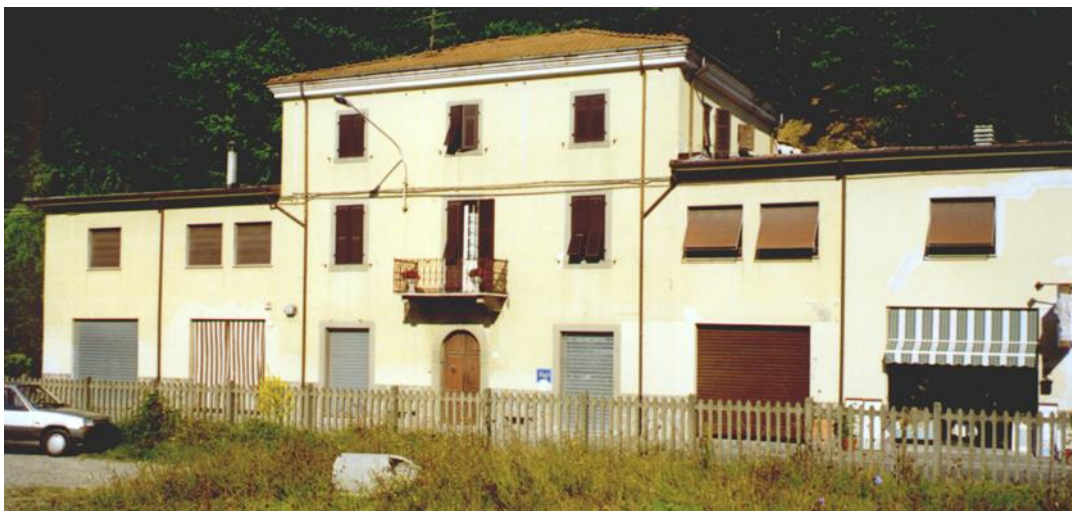
Figure 2. View of the building
