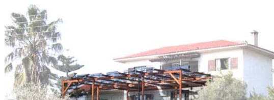
Figure 7: PV as shading element in the form of a solar pergola at CRES - Pikermi / GR (Photo: CRES).
