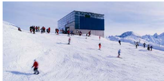
Figure 3: Façade integration of semi-transparent PV cell and PV module technology at the Kriegerhorn / AT (Photo: Sunways).
