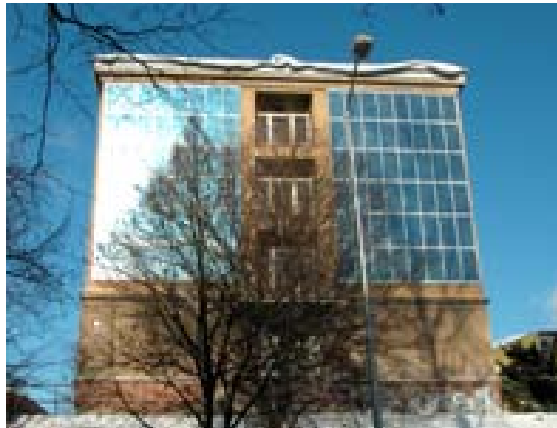
Figure 8: PV Façade with light blue solar cells manufactured by SOLARTEC for the University Liberec / CZ (Photo: SOLARTEC).
