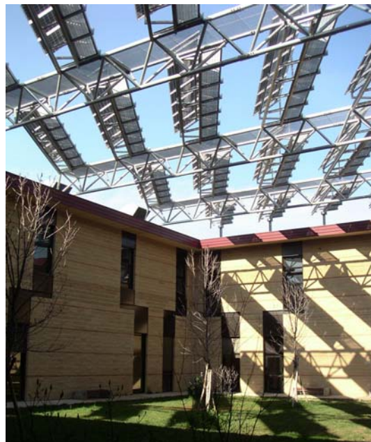
Figure 6: PV as shadowing element in the building envelope. University Florence - Sesto Fiorentino / IT (Photo: WIP).
