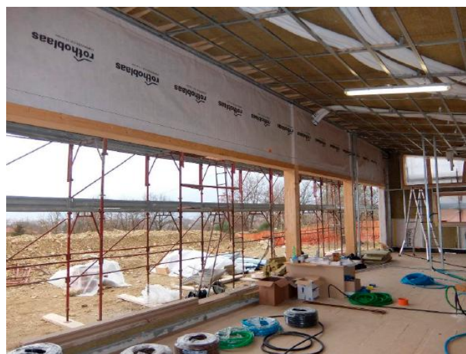
Figure 4. Living room of the building under construction.
