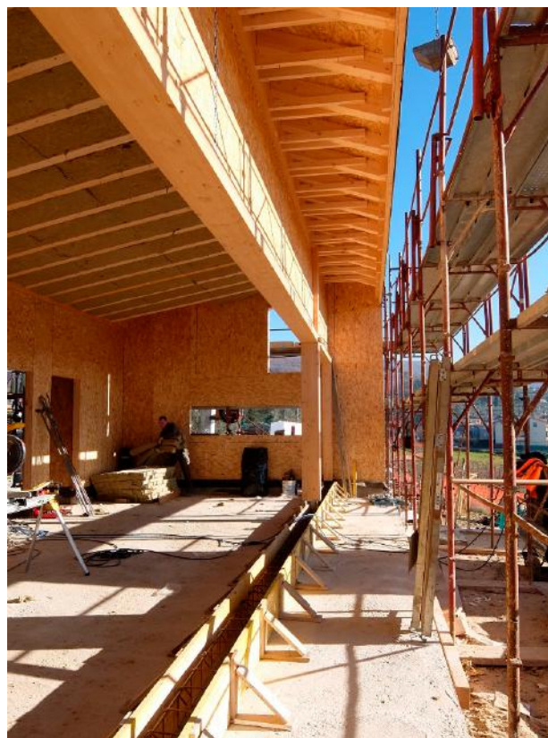
Figure 6. General view of the SW façade.
