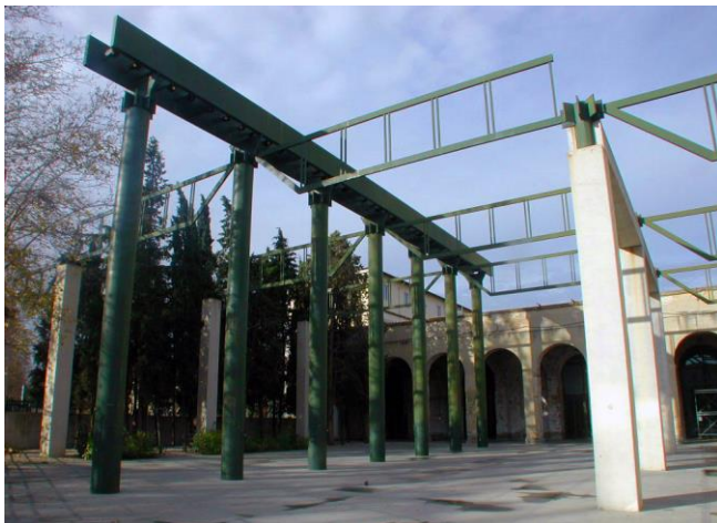
Fig. 11: The old Leopolda Station turned into a convention center (project by G. Aulenti, 1990)
