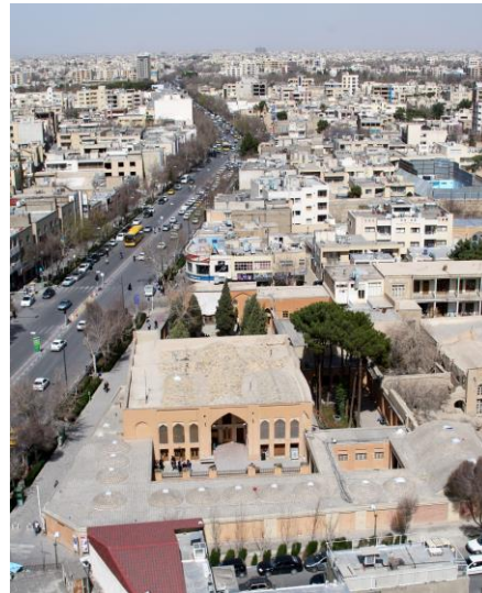
Fig. 5: Crossing the Hakim Nezami Street from inside of the historic fabric has led to fragmentation and destroying the territory of Julfa.
