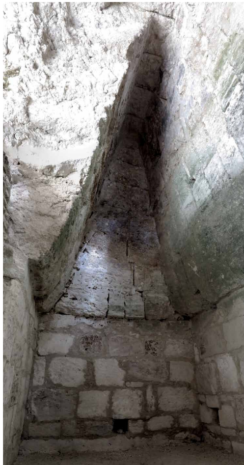
Figure 4. La Blanca, Palace 6J1, Room 2: high quality vaulted ceiling (Proyecto La Blanca, 2015)
