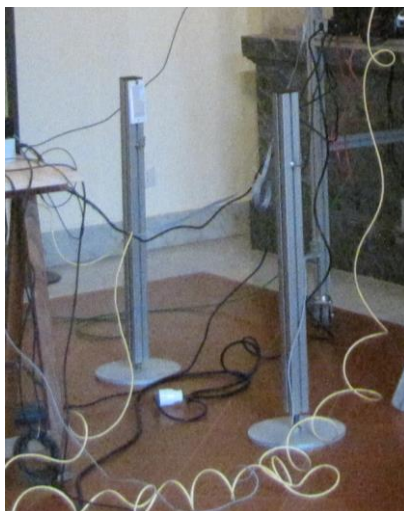
Figure 2.2. Image of the interlock system used to define the security area around the instrument
