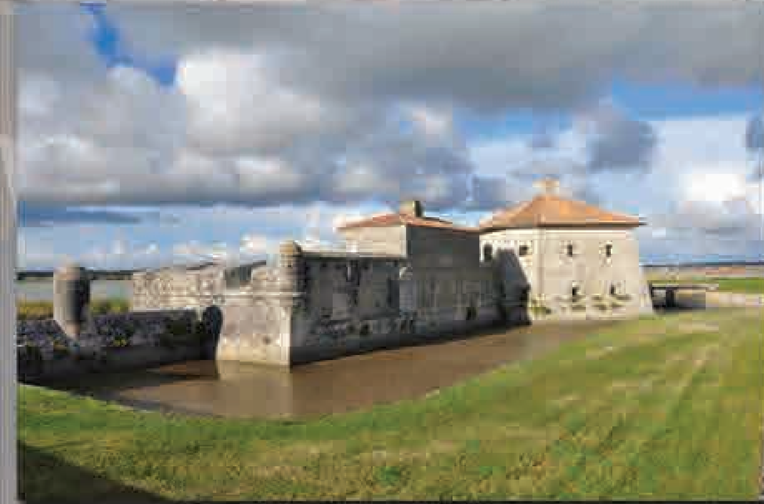
View from the west
