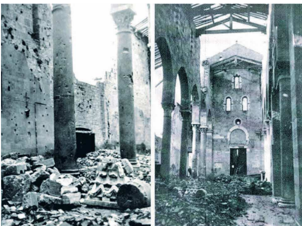
Fig. 2 – Damages due to bombing of 1943.
