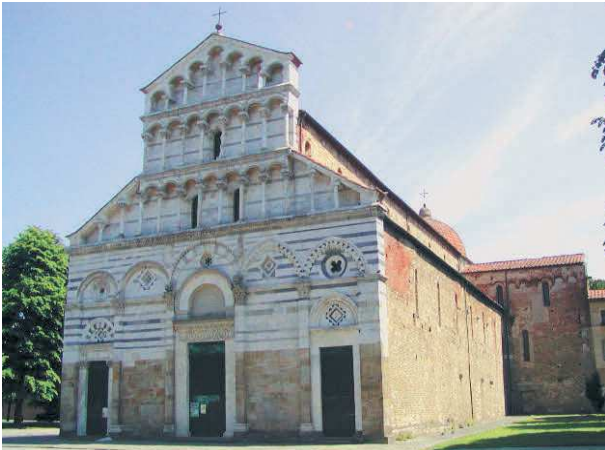
Fig. 1 – Facade of the Church of San Paolo a Ripa d'Arno in Pisa.
