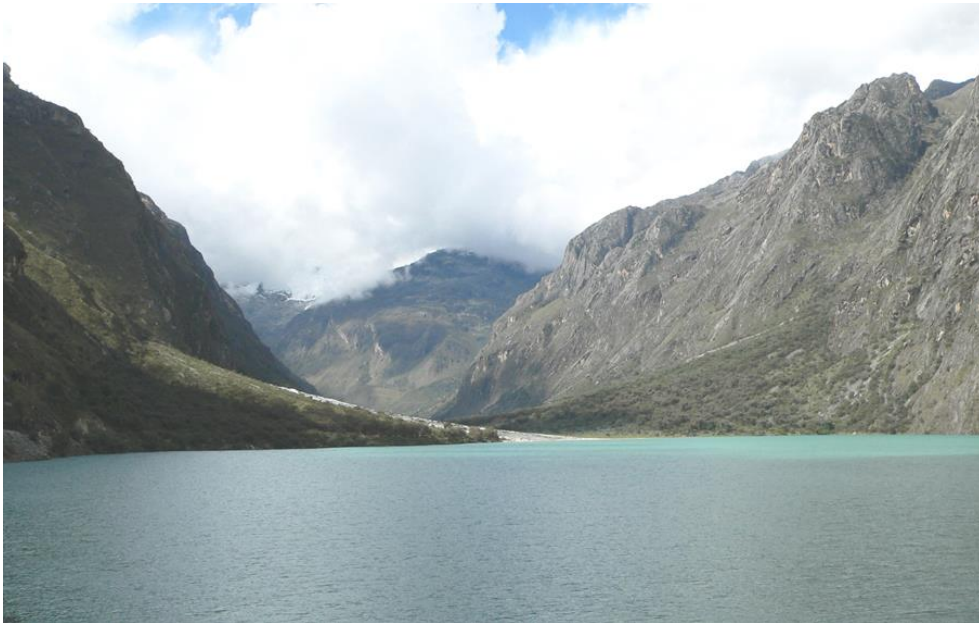
Figure 9 - View of Llanganuco Alto dam, Ancash Province, Peru.
