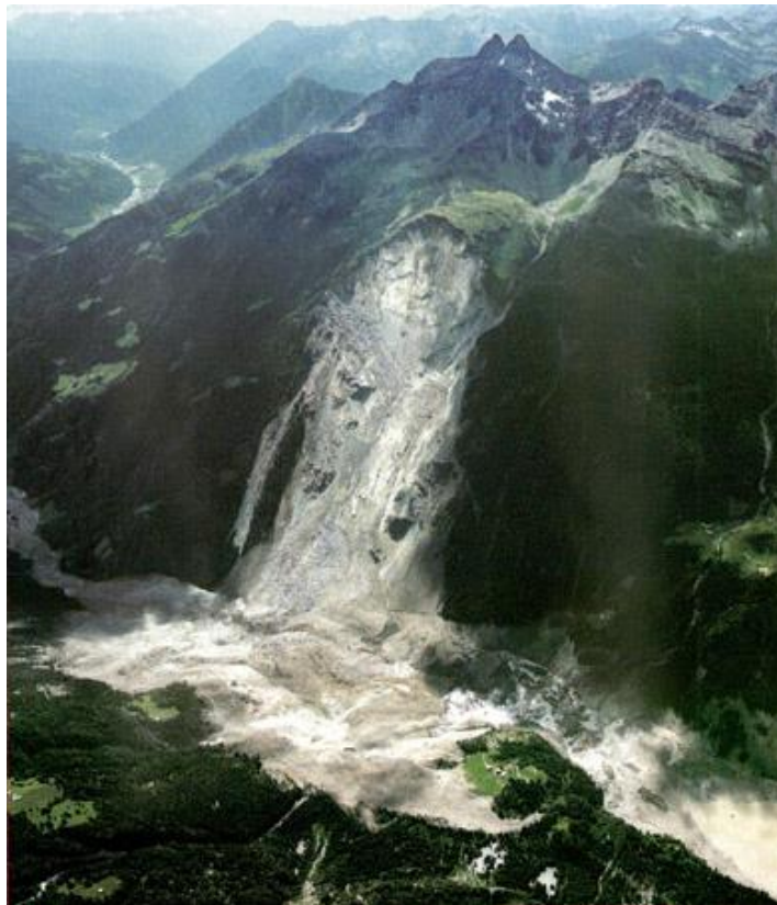
Figure 8 - Landslide dam of Val Pola, Sondrio, Italy, in 1987.
