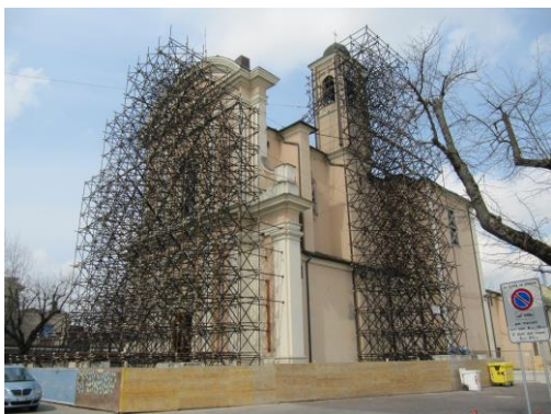
Figure 1. The church during restoration activity
