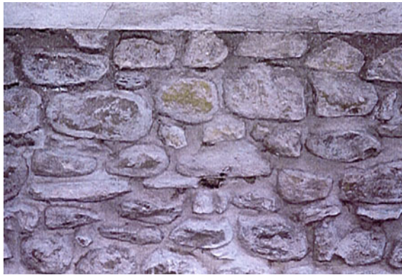
Fig. 23 View of the masonry texture
