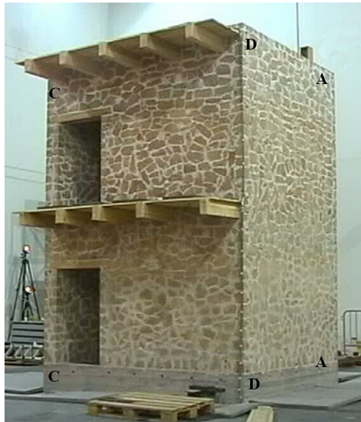
Figure 1. View of the unreinforced masonry (URM) prototype.
