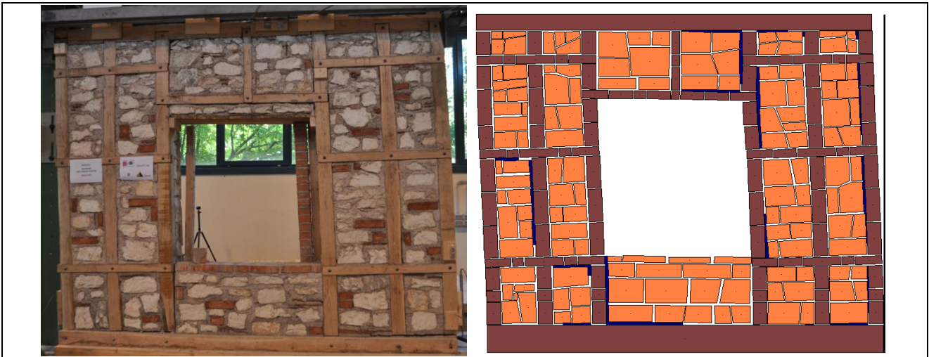
Figure 9. Ultimate deformed shape and cracking pattern. Comparison between experimental test and numerical modelling.
