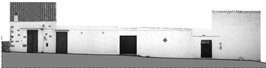
Figure 7. Northwestern facade from the road of Tanche (south-ern block), 2010 (Juan-Vidal & Merlo).
