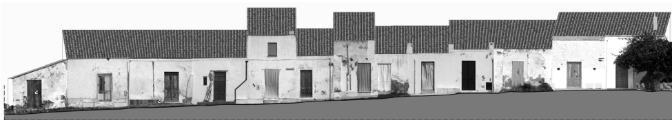
Figure 8. South-east facade from the road of Tanche (northern block), 2010 (Juan-Vidal & Merlo).
