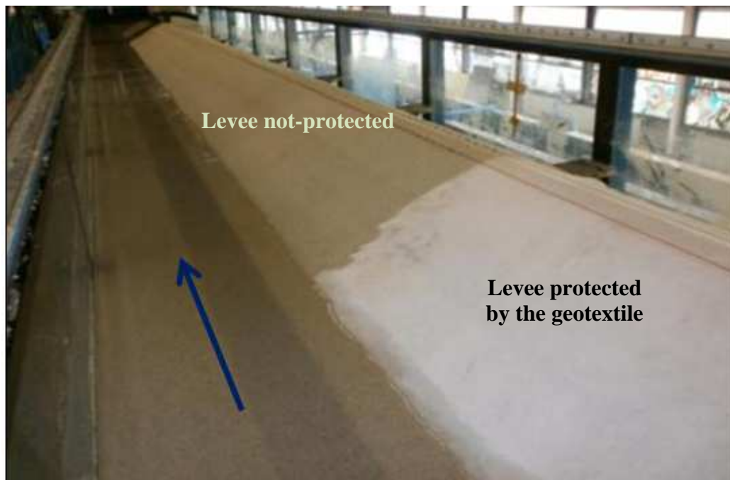
Figure 4.7: Geotextile protection of the levee.
