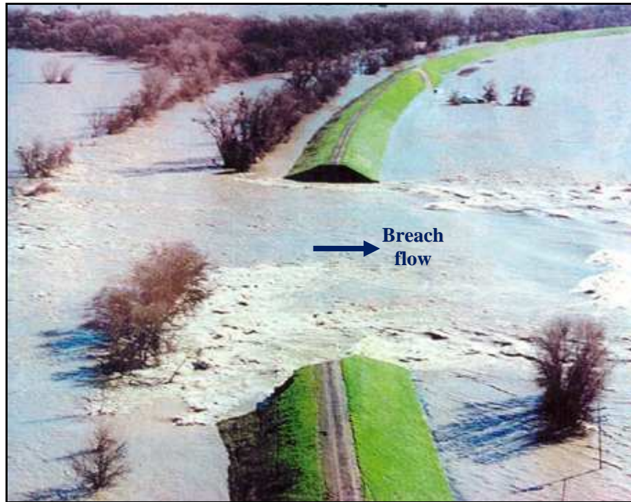
Figure 2.4: Californian levee (from Nagy and Tóth, 2005).
