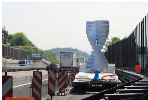
Figure 1.16: The in-field installation, from [16]
