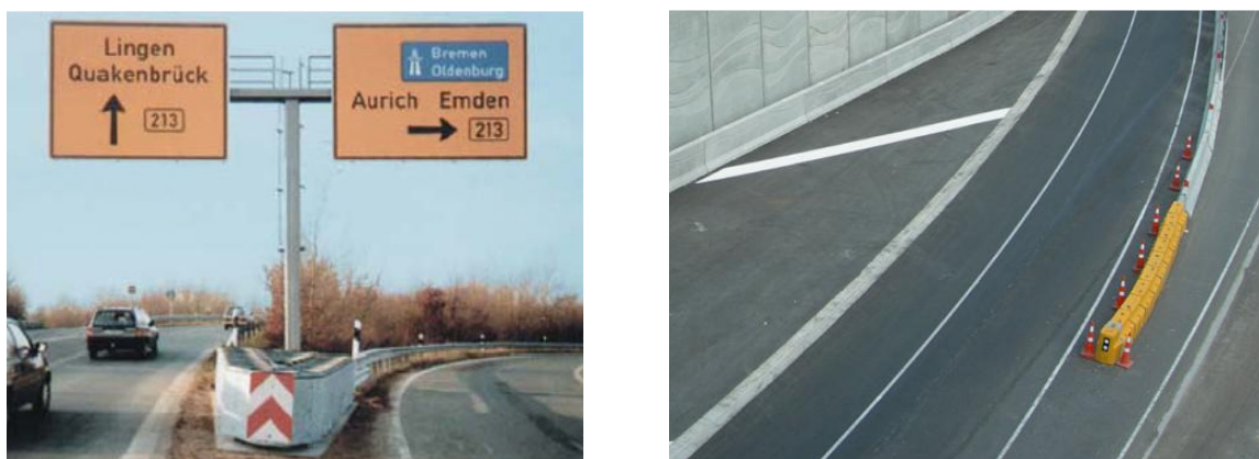
Figure 82: Examples of crash cushions (Sources: [A.2] and [A.51])
