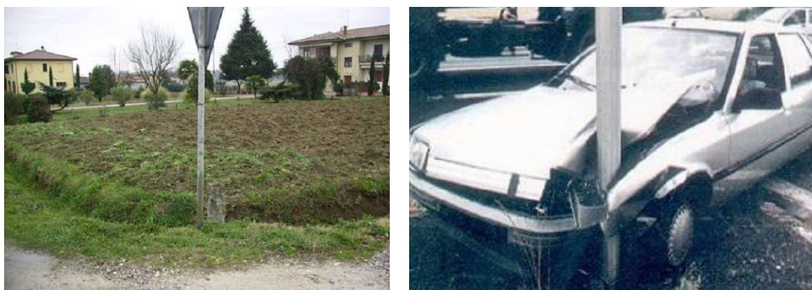
Figure 51: Examples of hazardous sign-posts (Source: [A.3])
