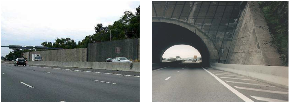
Figure 77: Examples of rigid median barriers [A.40]
