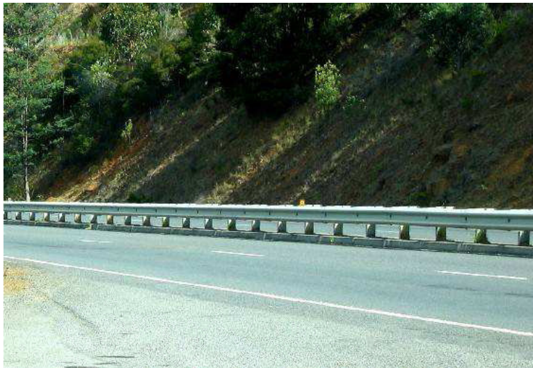
Figure 78: A typical median W-beam installation [A.40]
