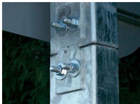
Figure 37: Breakaway/spliced pole ( left ) and slip base ( right ) [57]
