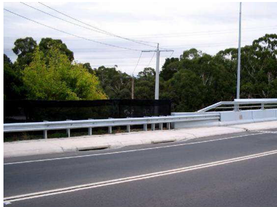
Figure 75: Transition between semi-rigid and rigid barrier [A.40]
