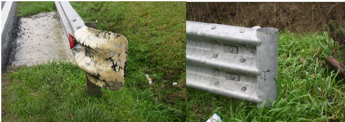
Figure 2: Unprotected (or 'exposed') terminals
