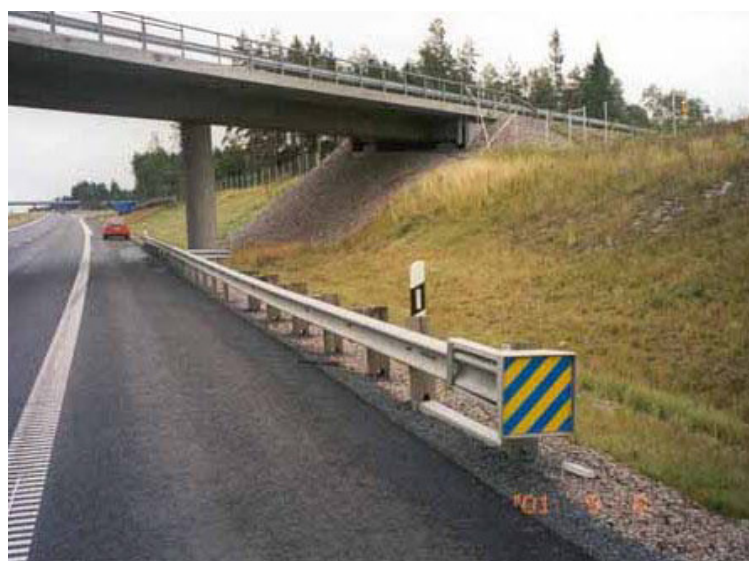
Figure 5: A tangent terminal [1]
