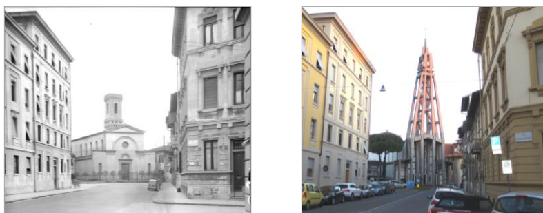
Figure 1: Views of the church in its original appearance and in its current conditions
