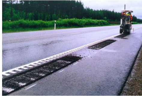
Fig. 6: Case study to evaluate the effectiveness of rumble strips on motorways in Sweden [4]
