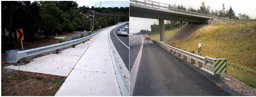
Fig. 3. Crashworthy barrier terminals ([5], left & [1] right)
