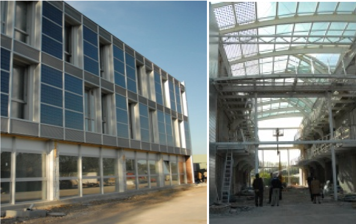
Figure 4. (a,) Details of the photovoltaic integrated facade. (b) Photovoltaic atrium integrated roof from inside
