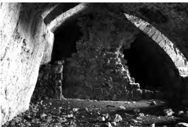
Fig 15 - Guest house: ground floor west view. (first room)
