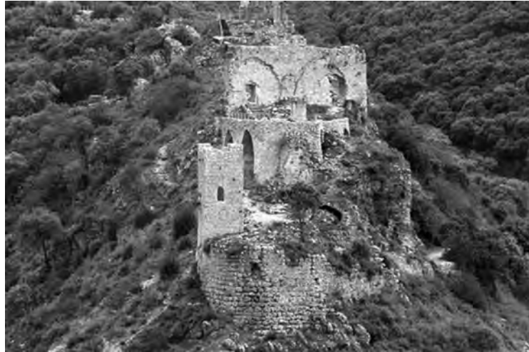
Fig 12 -View from west of Montfort castle, note the opening front along the lower end of the apparatus wall.
