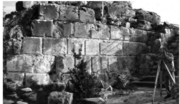
Fig 4 - Montfort: wall of the keep.
