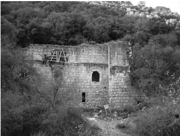
Fig 13 - Guest House: principal facade of the gothic building in the valley.
