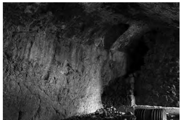
Fig 16 - Guest house: ground floor, detail of the rock wall with the vault.
