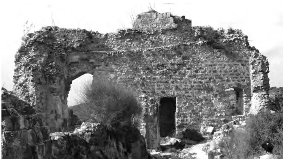
Fig 6 - Montfort: view from east of the north-south wall.
