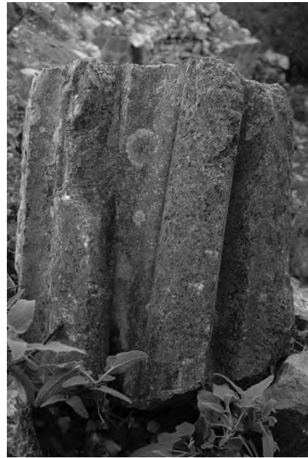
Fig 20 - Detail of an ashlar with almond-shaped ribs found on the top of the last vault.
