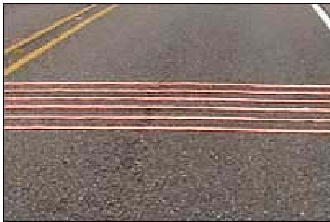
FIGURE 5 Raised transverse in-lane rumble strips.
