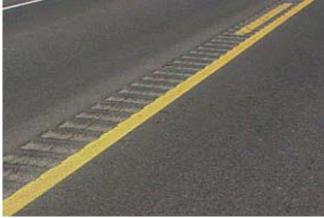
FIGURE 4 Centerline milled rumble strips.
